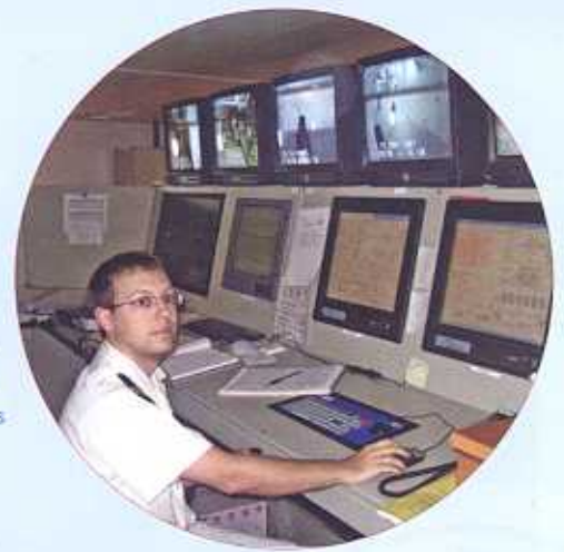
3rd A/E Christopher Ryals keeps a watchful eye in the engine control room monitoring critical systems throughout the ship.
